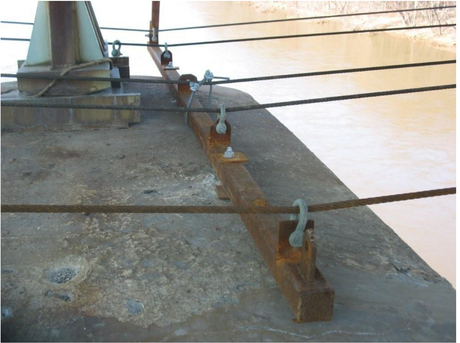
Main Cable System & Cable Hold Down Bracket
