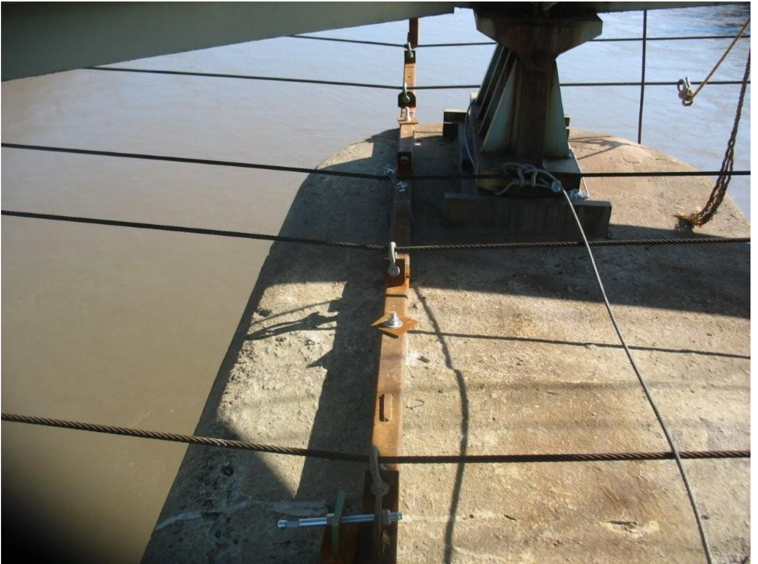
Main Cable System & Cable Hold Down Bracket
