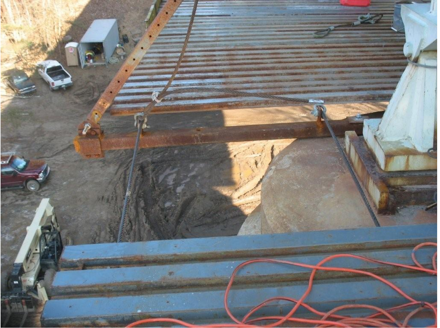
Cable Supported/Metal Deck Platform System & Cable Hold Down Bracket
