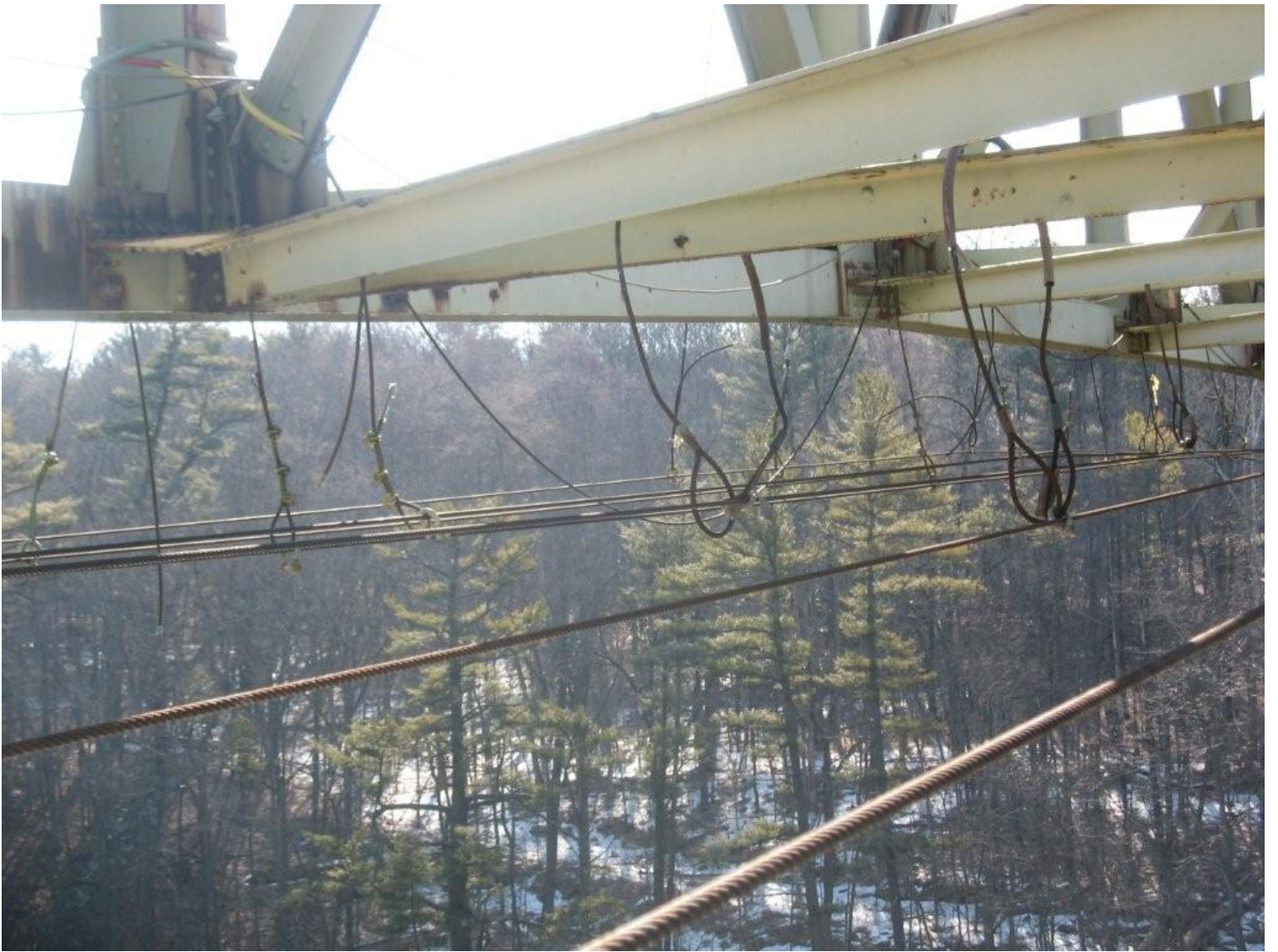
Main Cable System & Tie Up Supports
